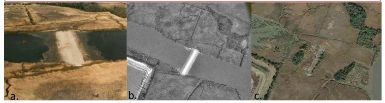
Images above illustrate a USACE closure at New Cut in the Savannah River Estuary. Closures will be constructed of rip rap and bedding stone, and will be tied into the marsh with sheet pile, similar to New Cut closure shortly after construction (a., b.). Wetland habitat is expected to fill in naturally on the low-energy side of the closures, as shown in c., approximately 20 years after construction of New Cut closure. (Figures 17, 18, 19 of USACE Feasibility Study Report, 2018)
