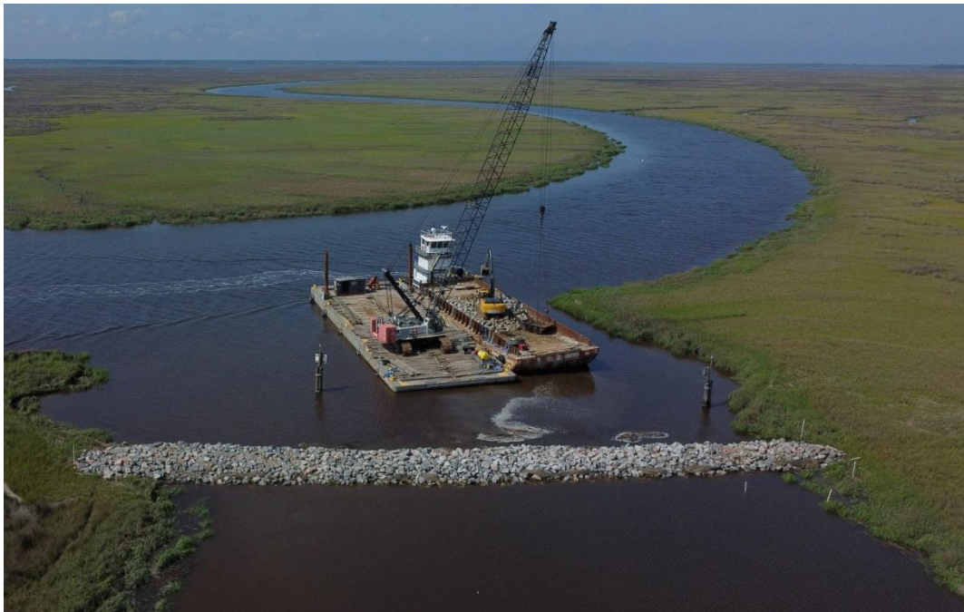
The Noyes Cut Restoration seen at Dynamite Cut.
